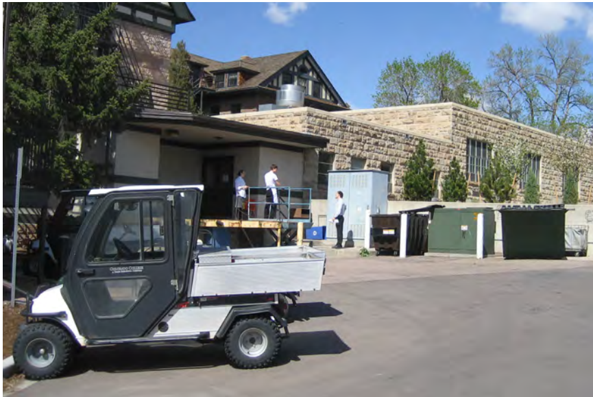
SERVICE AREA AT BEMIS HALL
