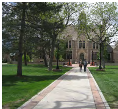
Cast-in-Place Concrete with Sandstone Bands
