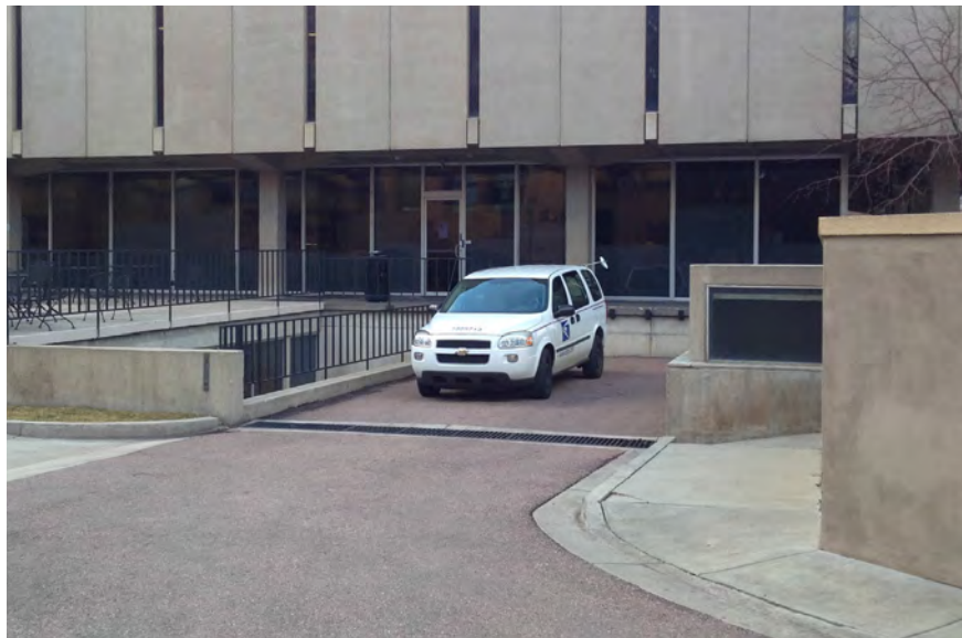
SERVICE AREA AT TUTT LIBRARY
