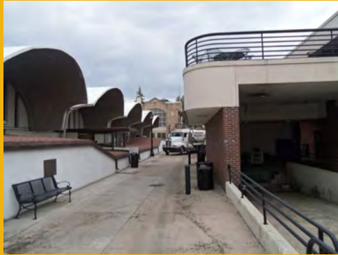
Service Alley at Honnen and Worner
