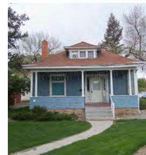
Cottages in Need of Renovation
