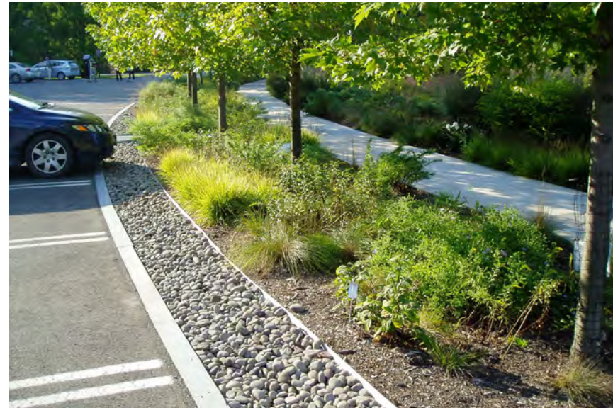
BIOFILTRATION STRIP, CORNELL PLANTATION
