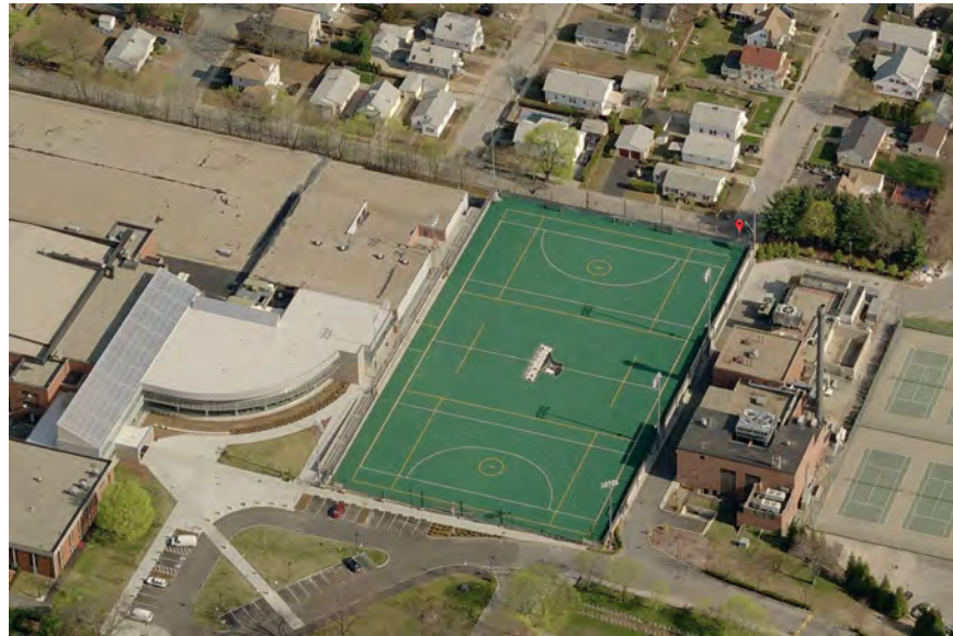
FIELD OVER UNDERGROUND PARKING GARAGE, PROVIDENCE COLLEGE
