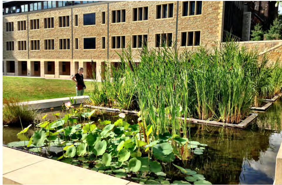
WATER FILTRATION, YALE SCHOOL OF FORESTRY & ENVIRONMENTAL STUDIES
