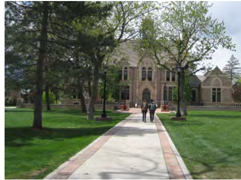
Cast-in-Place Concrete with Sandstone Bands
