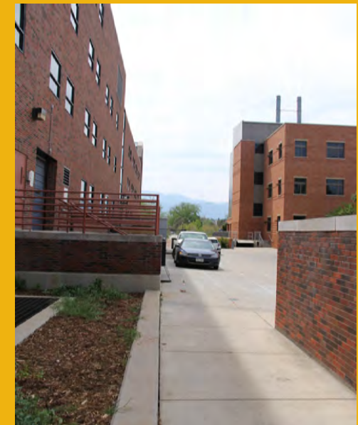
Service Access at Barnes Science
