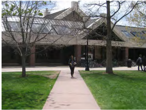
Cast-in-Place Concrete (Some are tinted to match adjacent building)
